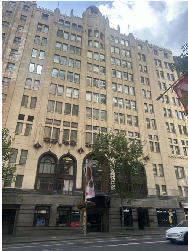
Figure 1: 60-70 Elizabeth Street, Sydney viewed from the east
